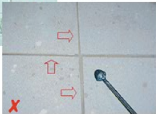
Inconsistent joint width
