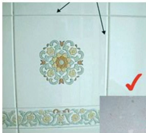
Consistent joint width
