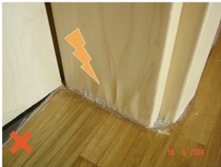
timber floor & door frame damaged
