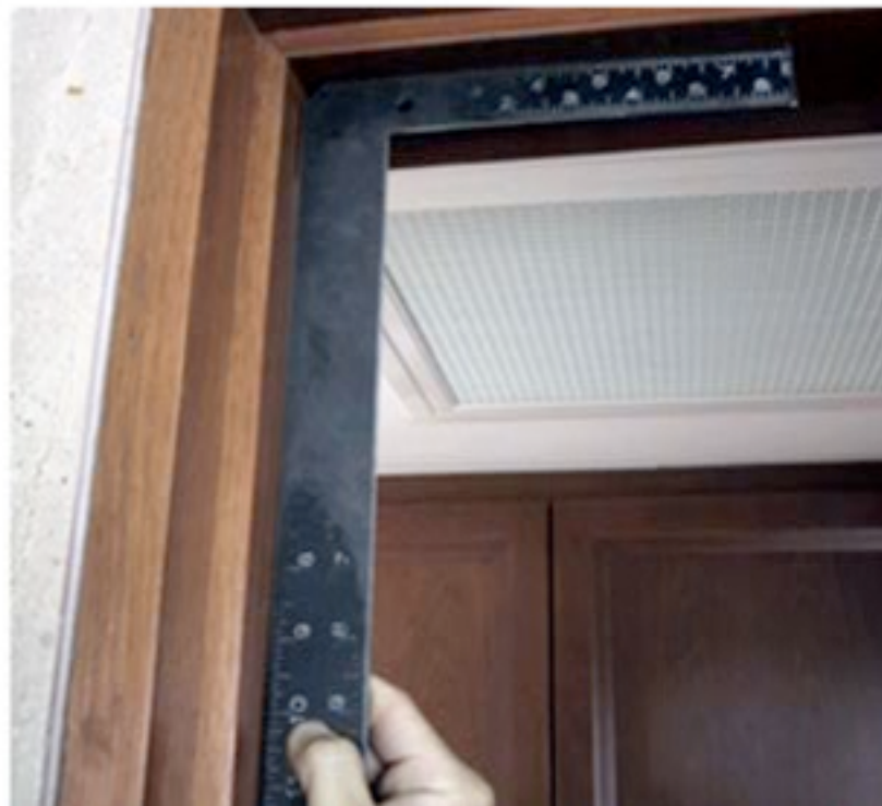
Door and frame corners maintained at right angles
